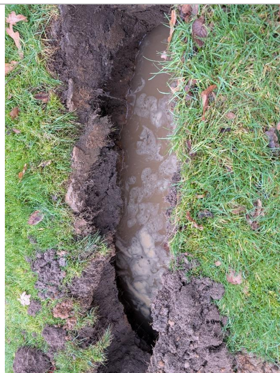
Figure 18. TP102 after 24hrs – note undermining of pit sides
